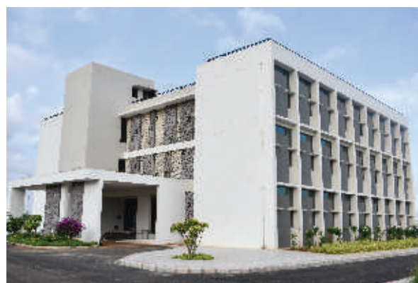
Aerial view of Additional Class Room Building (G+2)
