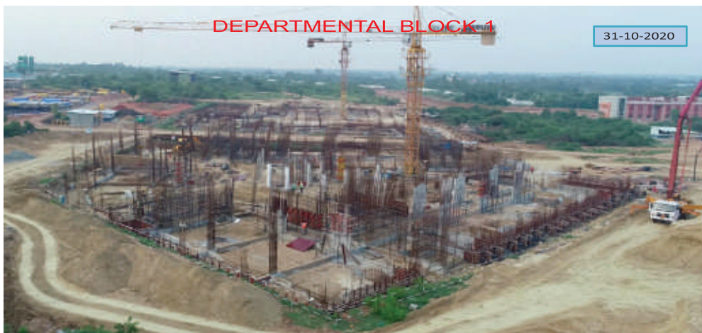
Department Block-1 construction in progress
