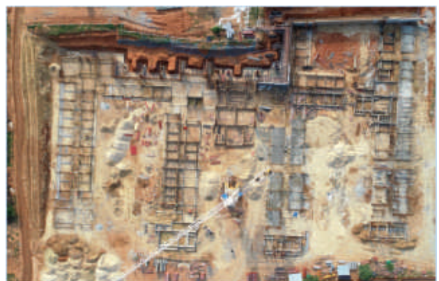
Hostel Block-1 construction at sit
